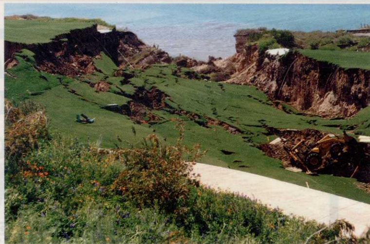
Holes 9, 12 and 18 at Ocean Trails were damaged in 1999 when a portion of the ledge on which they sat collapsed into the Pacific Ocean.
