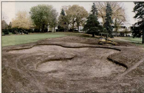
Bunker construction at Oak Ridge Country Club
