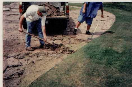
The old sod was shaved off and the top four to five inches of soil was dug out.
