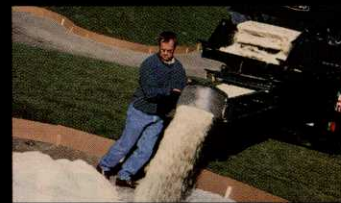
Cross conveyor with swivel action quickly fills bunkers and back fills trenches.
