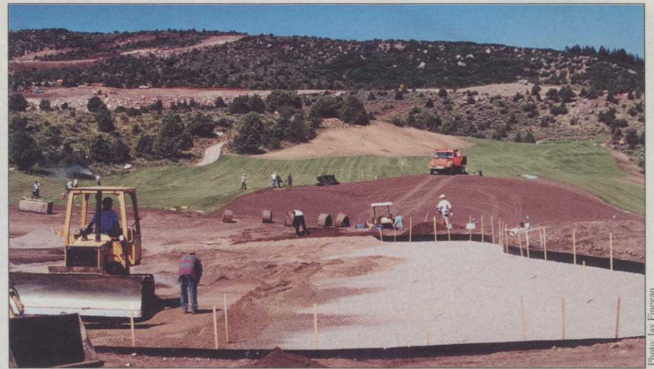
Workers laying bluegrass sod on the front nine of the Fazio Course at Red Sky
