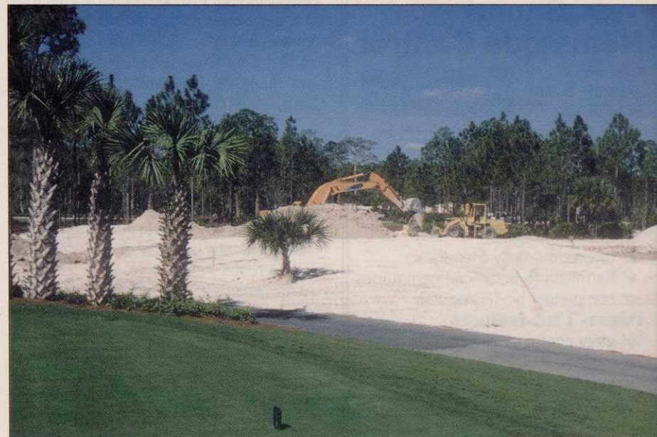
Construction is under way at the North Course at Mediterra.
