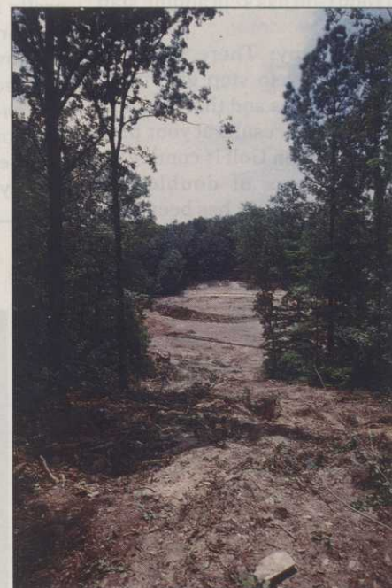
The 17th hole under construction at PTI's FarmLinks golf course
