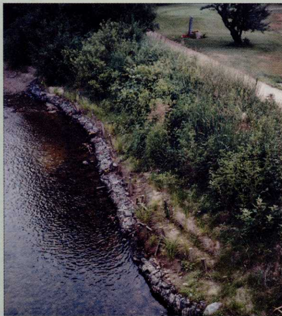
The stream bank restoration project unfolds along the 10th hole.
