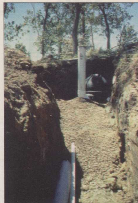
A SubAir vault unit partially backfilled.
