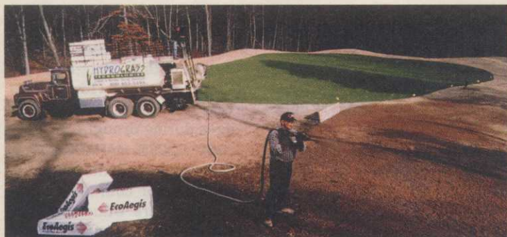
Hydrograssing near the 10th green at Blackstone National GC in Sutton, Mass.
