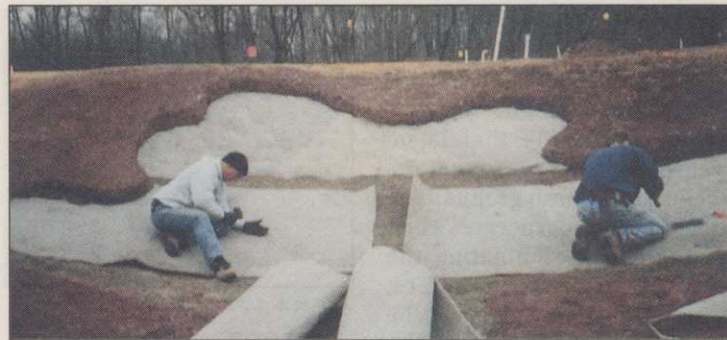
Bunker Woll uses natural fibers to control erosion.
