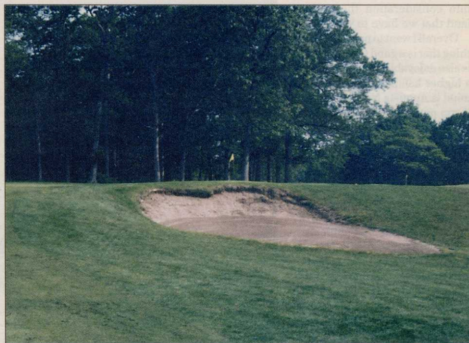
The Rulewich Group restored this greenside bunker on the par-4 4th hole at Yale University Golf Course. The bunker had eroded over the years, time "eating up" the slope. Rulewich installed 500 cubic yards of material and "flushed" the sand on the bunker.
