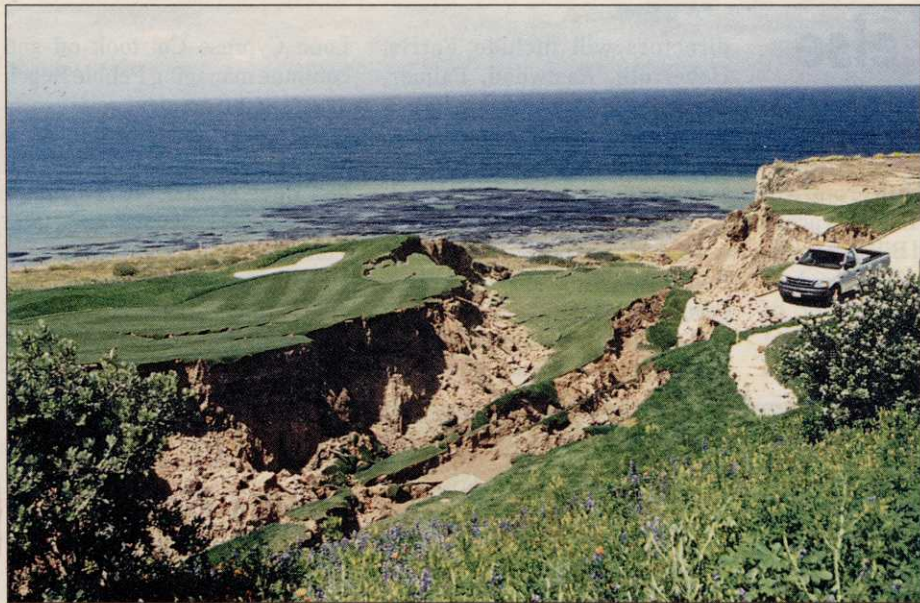
Developers of Ocean Trails Golf Course in Rancho Palos Verdes, Calif., are still seeking a solution to repair the landslide that pushed part of the 18th hole toward the ocean in early June.
