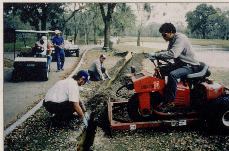
(Above) Roots pruned in 1996 at Riverside CC in Lake Jackson, Texas, show turf in the fairway and less on the tree side. (Below) Workers install a Biobarrier to prevent root encroachment at Riverside.
