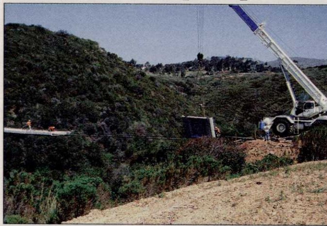
An FCI Constructors crew works on a stressed-ribbon bridge at The Bridges.
