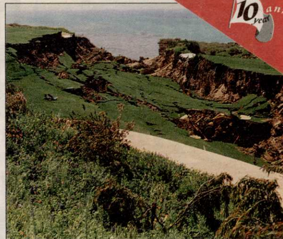
Ocean Trails Golf Course suffers landslide between the 12th and 18th fairways, losing a bulldozer into the chasm.
