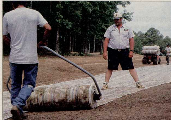
A crew lays down a roll of Z-Net with zoysiagrass implanted in it.
