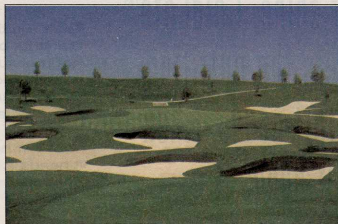
The Links at RiverLakes Ranch, an Environmental Golf facility under construction in Bakersfield, Calif.
