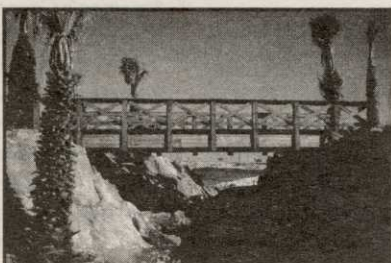
The Macho Combo: Combines the beauty of wood and the strength of maintenance free self-weathering steel. Bridge designed by Golf Dimensions.
