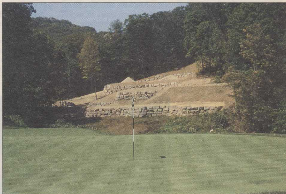
Limestone boulders formed walls and served as the foundation for tees and greens at aptly named Olde Stonewall Golf Club outside Pittsburgh. This shot of the par-3 15th hole looks back from the green at four sets of tees in the background.
