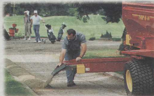
Backfill ditchlines, build cart paths, or place wood chips and compost around trees, plants and in flower beds. The cross conveyor can move in any direction.
