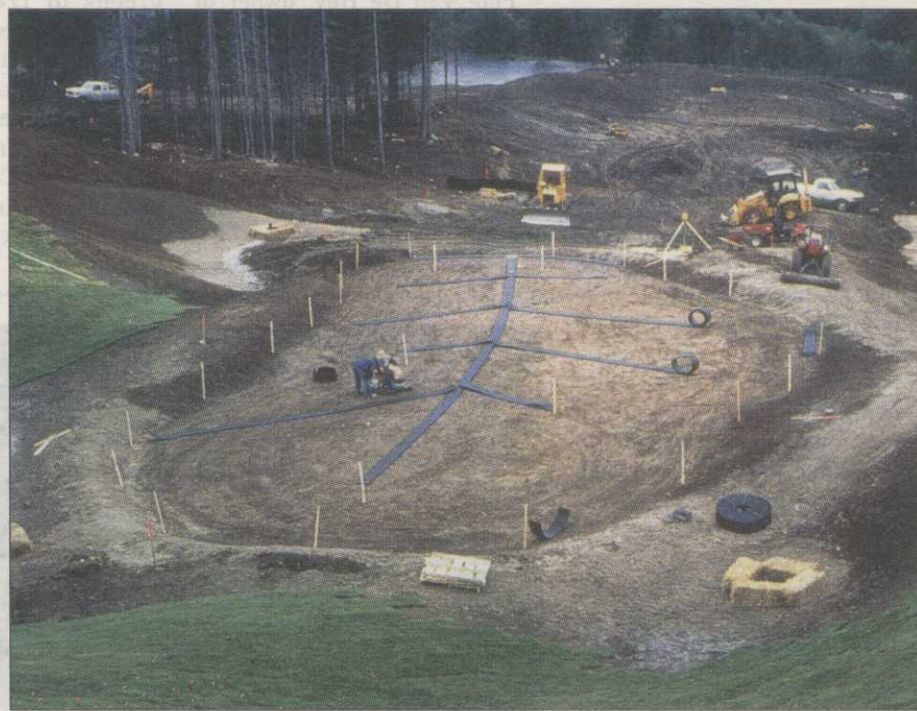
One of the earlier Hurdzan-Fry greens showing ADS AdvanEDGE pipe installed horizontally on the sub-base.
