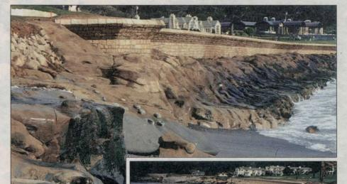
The concrete abutment, at right, during construction of the new seawall along the 18th fairway of Pebble Beach Golf Links. The final version is shown above at low tide.
