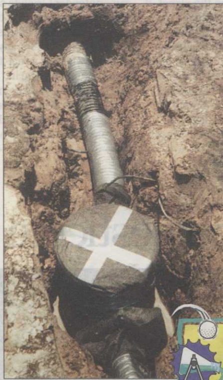
"X" marks the spot where the drainage grate is covered with a geotextile filter cloth.
