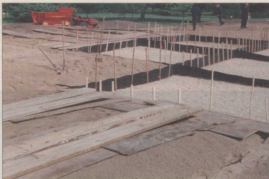
Root-zone mix cells at for turfgrass testing at North Shore Country Club. All the work is done by hand, ensuring no cross-contamination. The barriers, from pea gravel to the top, are permanent.
