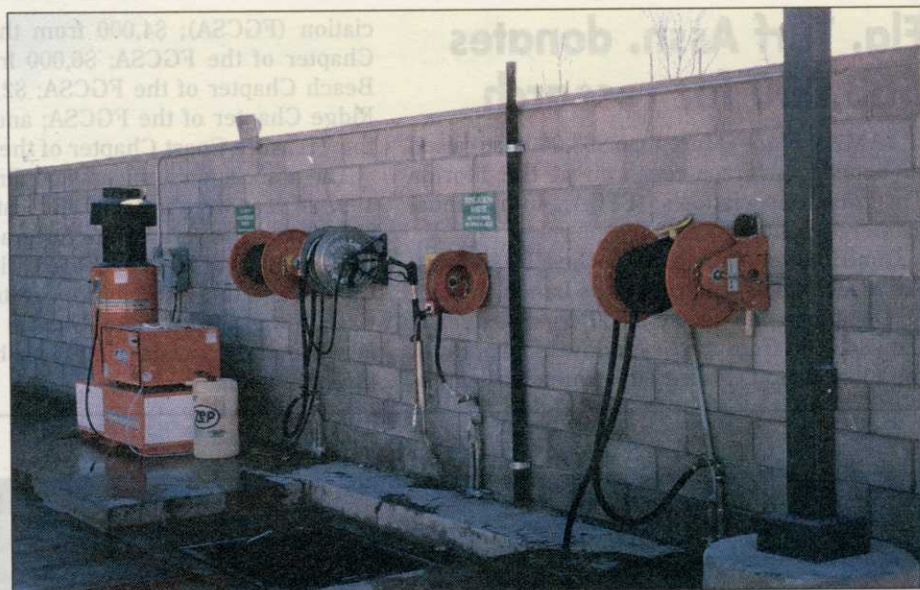
The state-of-the-art, environmentally friendly wash rack at The TPC at The Canyons, designed with efficiency in mind.
