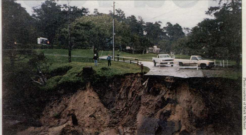
Access to the 15th tee at Pebble Beach Golf Links is destroyed as a result of the El Niño-driven storms in early February.
