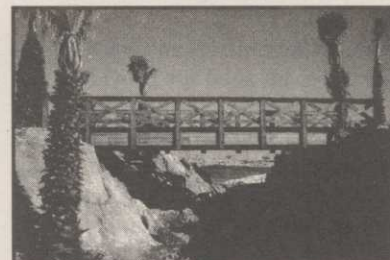
The Macho Combo: Combines the beauty of wood and the strength of maintenance free self-weathering steel. Bridge designed by Golf Dimensions.
