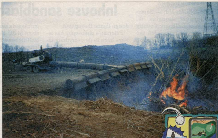
A blower helps a crew keep smoke to a minimum after clearing brush on a golf course.
