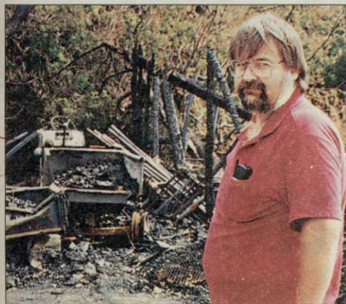
INTO THE BREACH When fire ravaged the maintenance facility at South Hills Country Club in Franksville, Wis., superintendent John Syty received a huge helping hand. See page 49.
