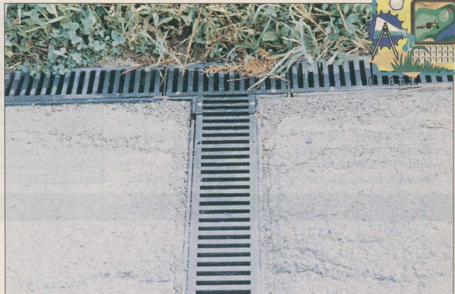
An effective way to help alleviate the problems associated with heavy rains over cart paths.
