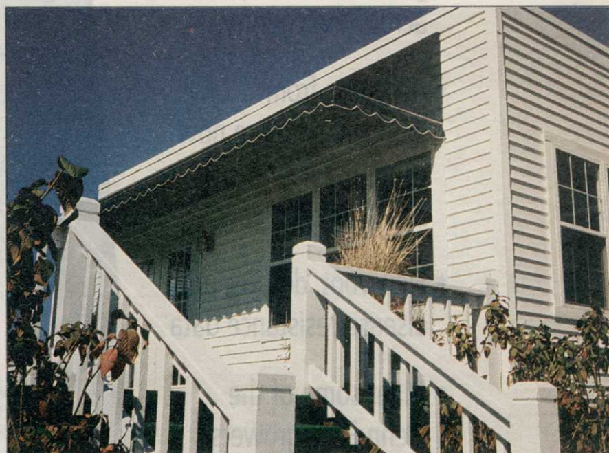
Temporary clubhouses don't have to be unsightly trailers sitting starkly in parking lots. To wit, this clubhouse facility at Hamilton Golf Club in Fishers, Ind.
