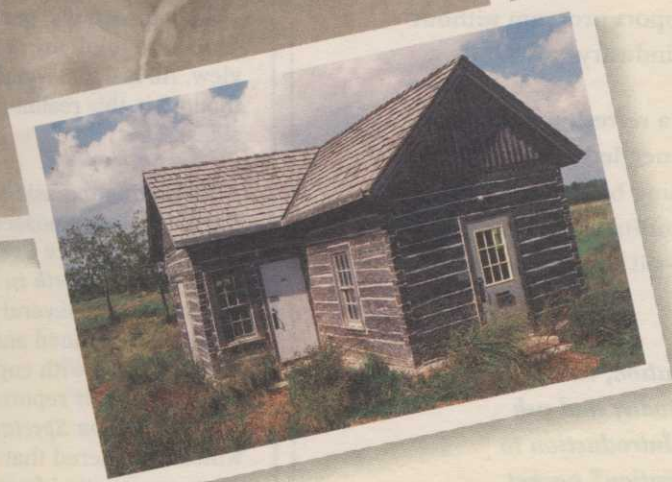
This Norwegian farm building was disassembled, numbered, and shipped to Blackwolf Run to serve as a rest station.
