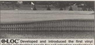
plastic interlocking panels for soil retention applications
