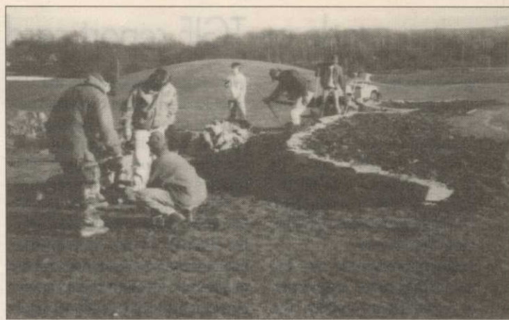
Students build a retaining wall at one of 10 sites on Penn State's newly redesigned Blue Course.
