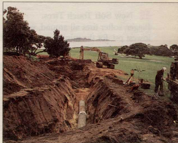
Effluent pipe is laid along the 14th fairway at Pebble Beach Golf Links.
