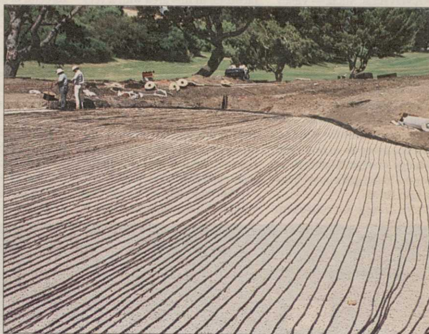
The 4th green at Palos Verdes Country Club, now equipped with the TurfTemp system.
