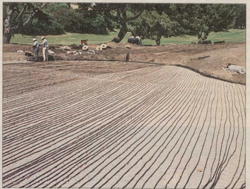
The 4th green at Palos Verdes Country Club, now equipped with the TurfTemp system.
