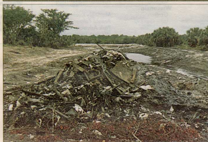
Heavy, metal trash filled the St. Lucie County landfill, left, before Guettler & Sons and architect Jim Fazio turned the site into Fairwinds Golf Course, above.
