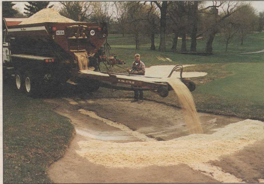
After the bunkers at Scioto Country Club were totally renovated, The Placer installed sand at an initial six-inch depth on the bottoms and two to three inches on the slopes with minimal handwork.
