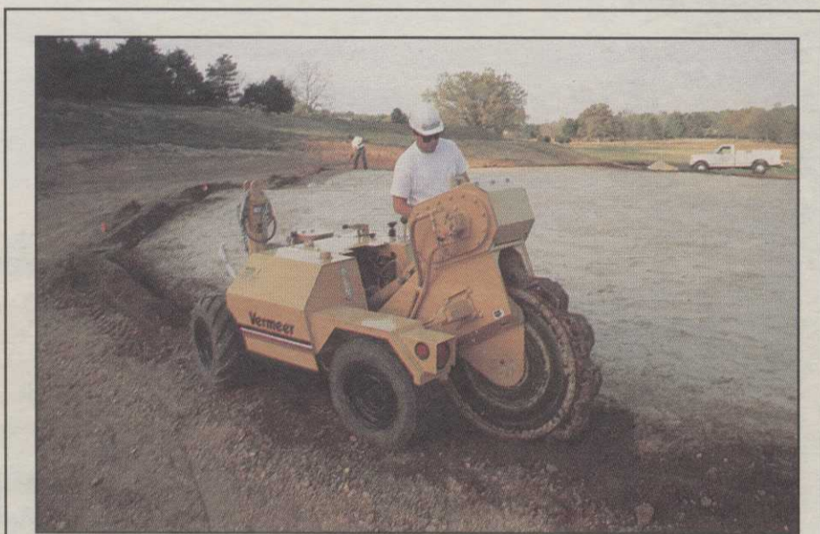
LAYING THE GROUNDWORK
