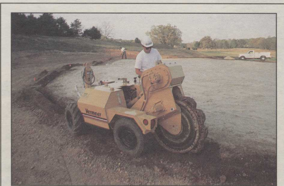
LAYING THE GROUNDWORK
