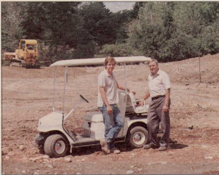
Gordon Bliss, right, and his son Kevin take a look at the construction at Blissful Meadows Golf Club in Uxbridge, Mass.
