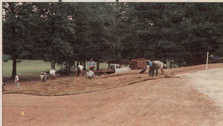
A crew from Chantilly Turf Farms, Inc. lays bluegrass sod on the perimeter of the 13th green at International Town and Country Club. Chantilly, a subcontractor to John Ponko Inc., will put down bentgrass sod on the greens. Chantilly grew the bluegrass sod, while Summit Hall Turf Farm grew the bentgrass.
