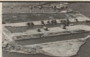
Seawall installation for waterfront development. Pointe Fourchon, LA.
