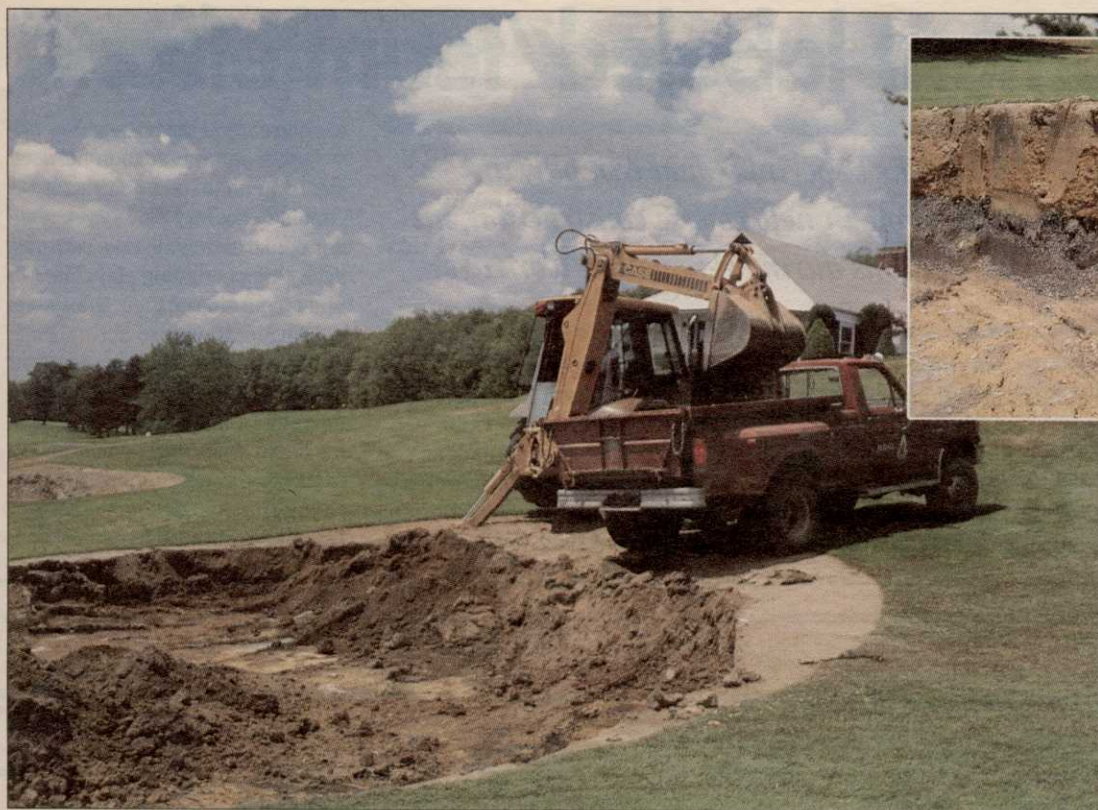
Photos courtesy of Aspen Corp. An Aspen Corp. backhoe operator uses extraordinary care as he digs out a sand bunker at Wyoming Valley Country Club in Wilkes-Barre, Pa. The inset at top right shows the layers of sand, ash and soil that had been added to the original bunker when A.W. Tillinghast remodeled the original nine holes and added a new nine in 1924.
