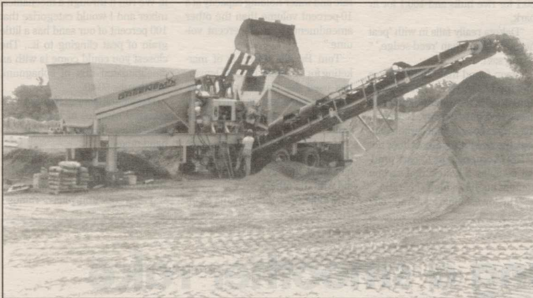
A blender sends a predetermined mix into a stockpile
