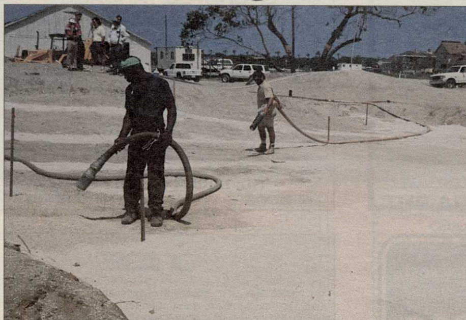
Green sandscaping allows workers, left, to apply a four-inch gravel layer to a new green. The truck, above, transports gravel and pumps it to the site.
