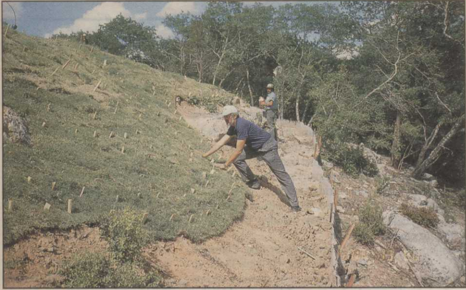
A worker installs prairie buffalograss alongside a bunker at the 17th hole of the new Ben Crenshaw-designed course at Barton Creek Country Club in Austin, Texas. This Texas A&M-developed buffalograss is one of the new semi-arid grasses being developed around the
