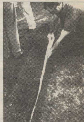
Lesco subsurface drainage system
